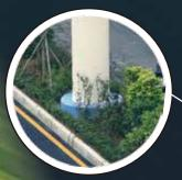
The pillars that support the single track beams are approximately 1 m (3.5 ft) in diameter and can be constructed in the medians of existing roads.
